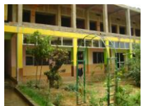
outside view of the play hall/ on going construction
